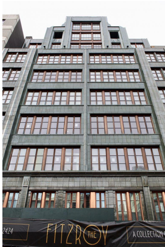
The northern elevation of The Fitzroy at 514 West 24th Street. Photo by Michael Young
